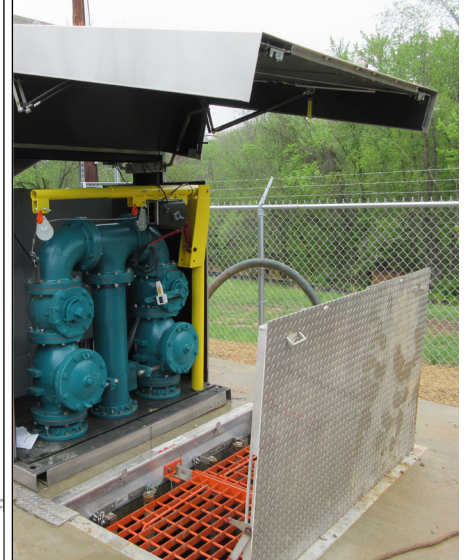
Hatch with Safety Grate in a NoVault™ Pump Station
