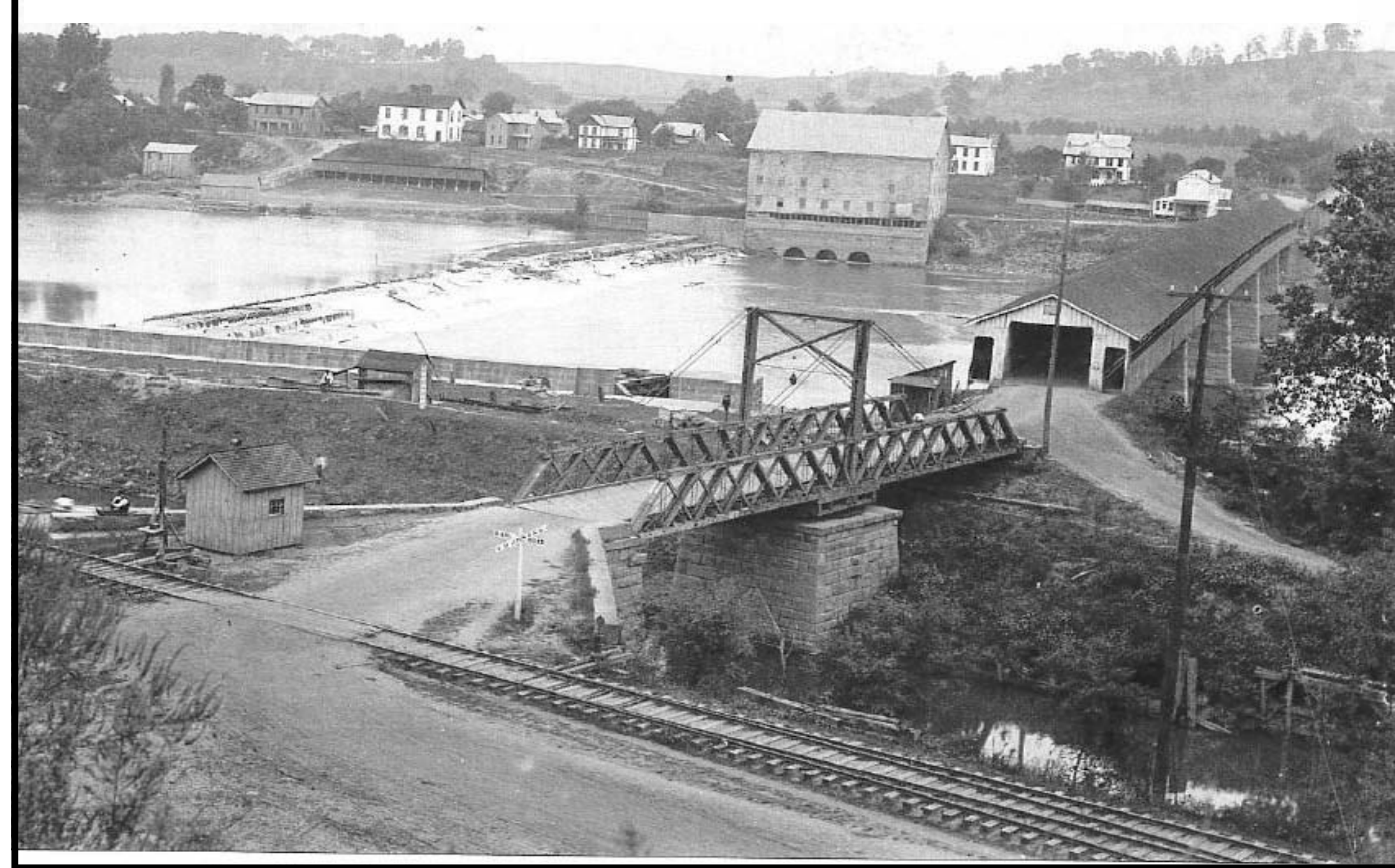
Covered Bridge with swing span
