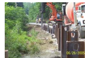
Old River Road CR6, embankment repair
