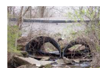
Sally Road Bridge, before replacement
