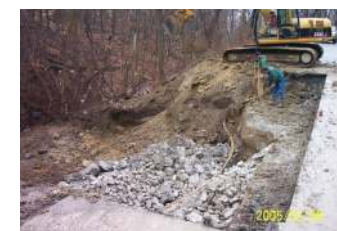
Richvale Road CR3, during repair
