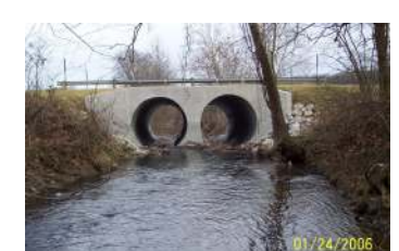
Sally Road Bridge, new culverts and headwalls
