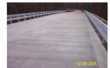
Pleasant Valley Road, bridge after repair
