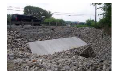
N River Road CR3, after repair
