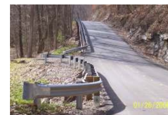
Old River Road CR6, after repair
