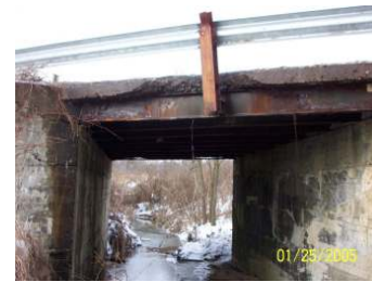
Shannon Rd old bridge removed
