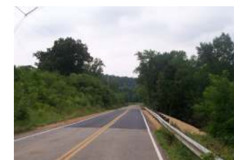
Shannon Road CR48, after repair
