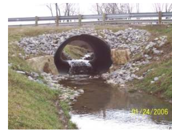
Shannon Rd new culvert installed
