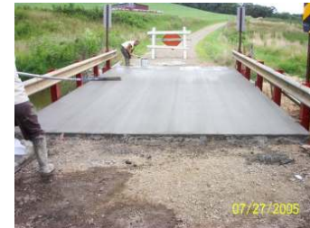
North Branch Rd after repair
