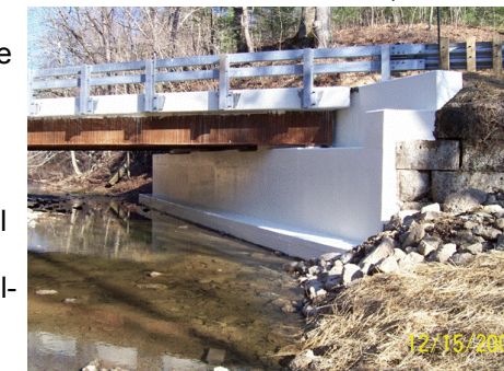
Cutler Lake Rd #6031-293 After Replacement
