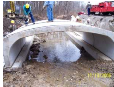
Coopermill Rd during construction
