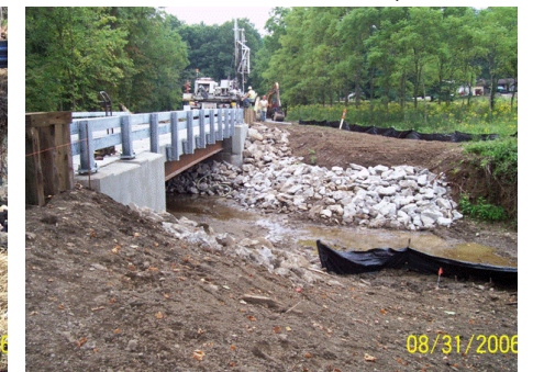
Cutler Lake Rd #6031-269 After Replacement
