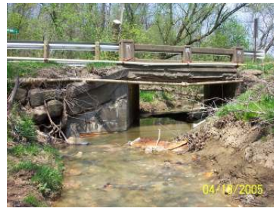
Coopermill Rd before construction
