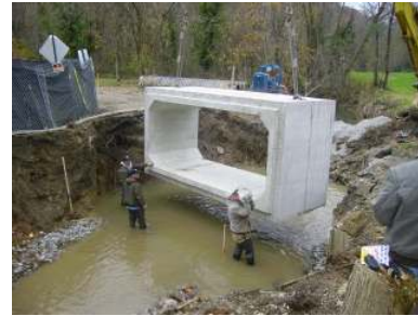
Woody Ln during construction
