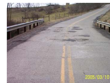
Existing Clay Pike Bridge
