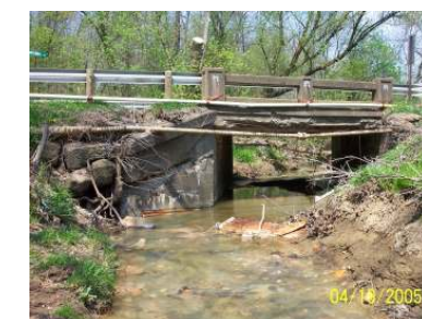
Existing Coopermill Rd Bridge
