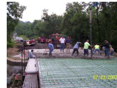
Clay Pike bridge in construction
