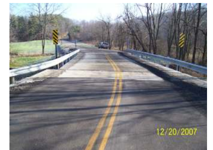
Clay Pike bridge after replacement
