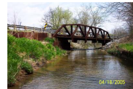
Coopermill Rd. in Springfield Township CR71
