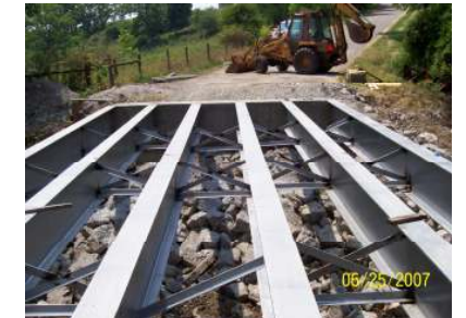
Clay Pike bridge in construction
