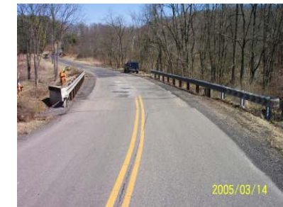
Clay Pike bridge before replacement
