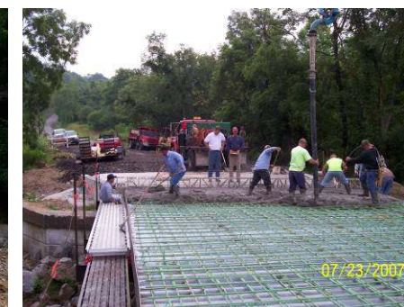
New reinforced concrete deck poured
