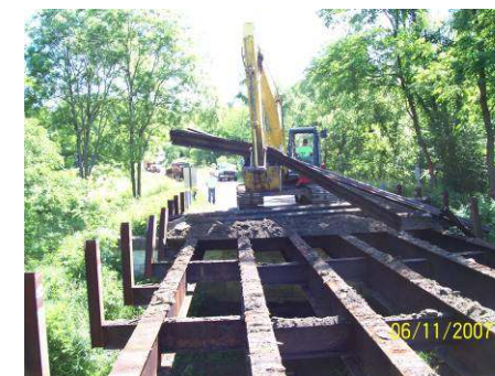
Bridge deck being removed
