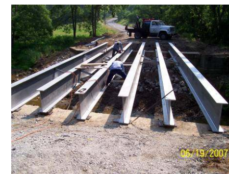
New steel beams set in place
