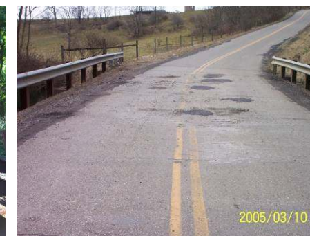
Existing asphalt deck
