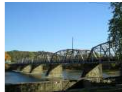
The Philo/Duncan Falls bridge spanning the Muskingum River
