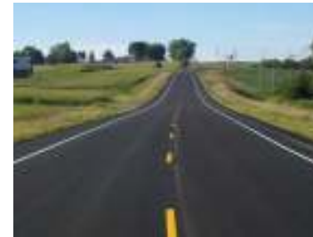
A view of North Pointe Road completed; view to Richvale Road
