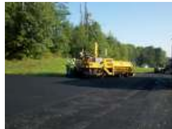
Paving crew resurfacing North Pointe Road at Powelson Road
