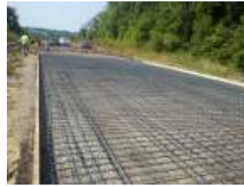
Forms complete and ready for concrete over Vista View Drive
