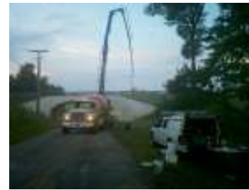
Concrete pump truck pouring the concrete on North Pointe Road
