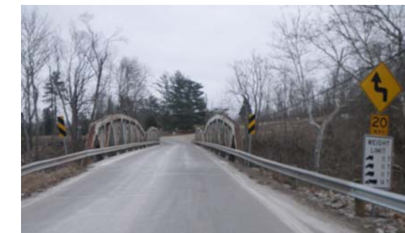
SR555/Old River Rd Bridge (at Grantcliff Rd)
